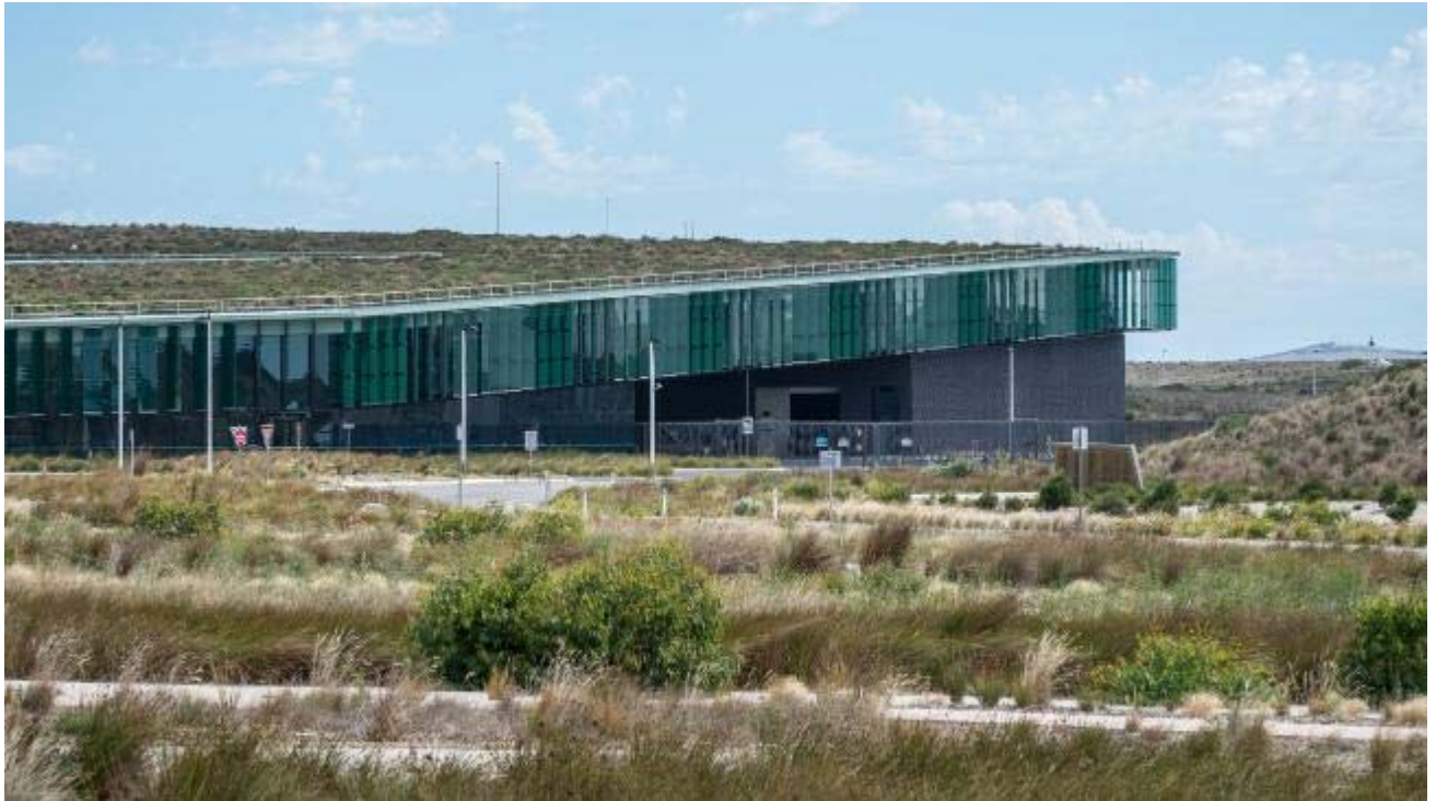
Victoria's desalination plant remains in mothballs, a monument to our stupidity. Picture: Jake Nowakowski
