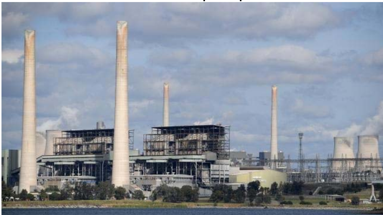
Liddell power station in Muswellbrook in the NSW Hunter Valley. Picture: AAP
