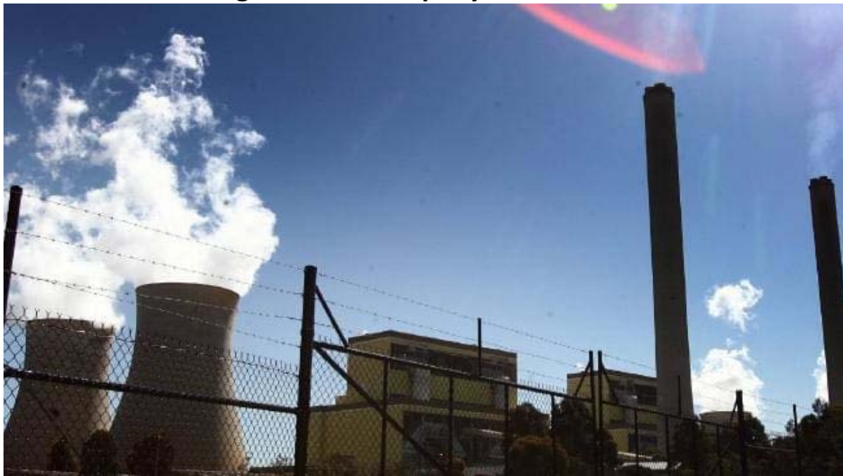
The Loy Yang power station in West Gippsland in Victoria.
