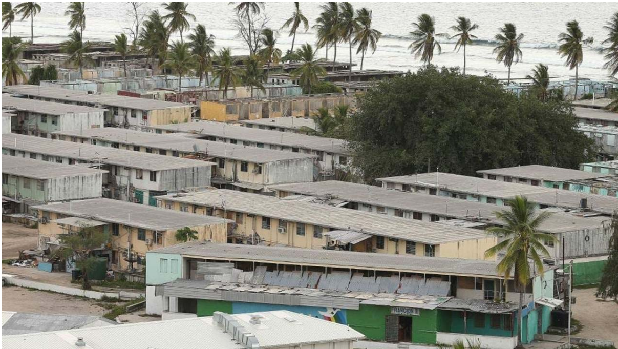
Old concrete workers flats on Nauru. Picture: Lyndon Mechielsen
